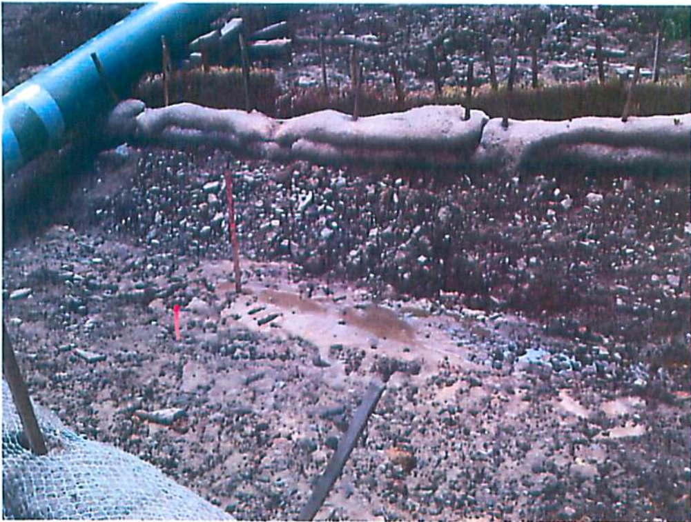
Photo 8. M3 stream crossing of Jake Run in Monongalia County.
