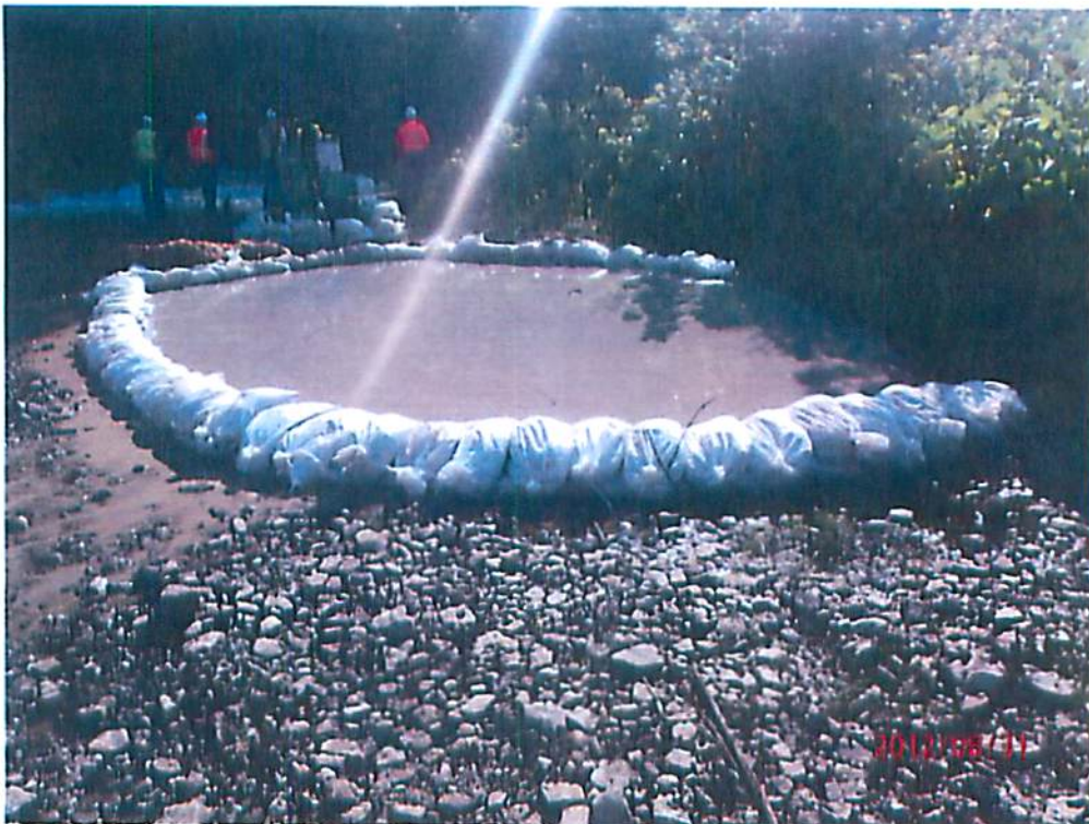
Photo 14. Containment around inadvertent release on Dunkard Creek.
