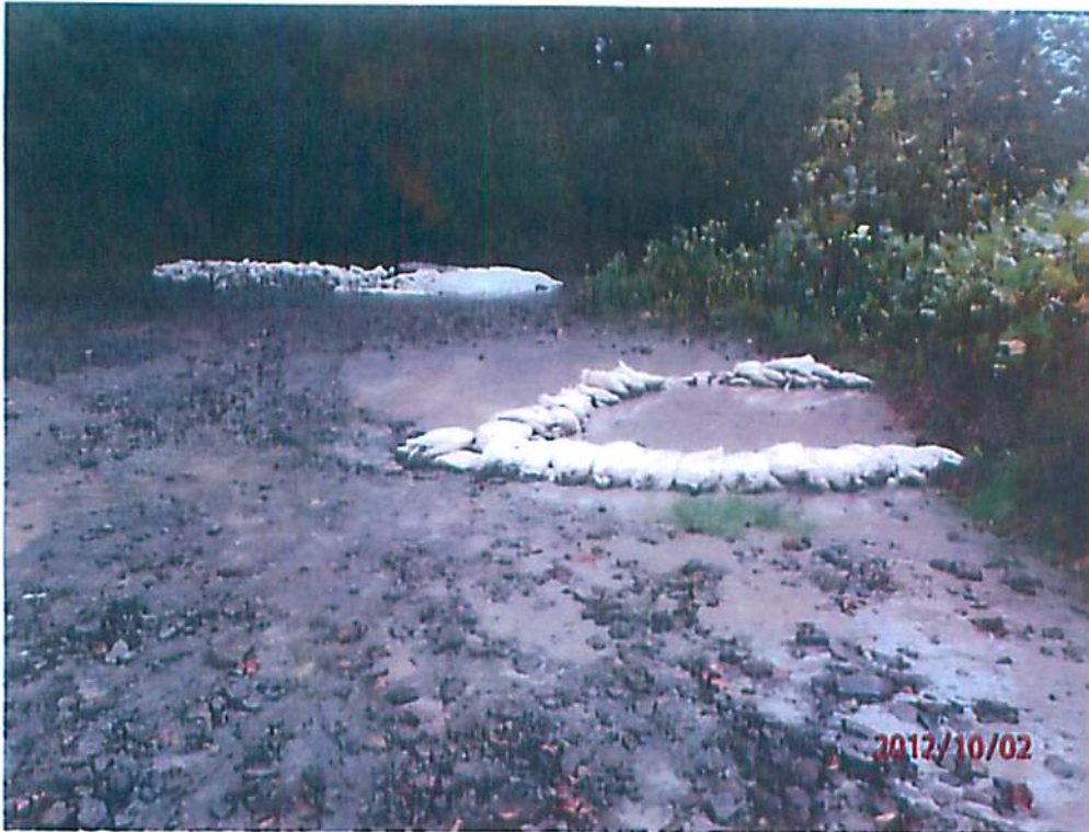
Photo 19. Original containment area for inadvertent release into Dunkard Creek (shown at date of second release).
