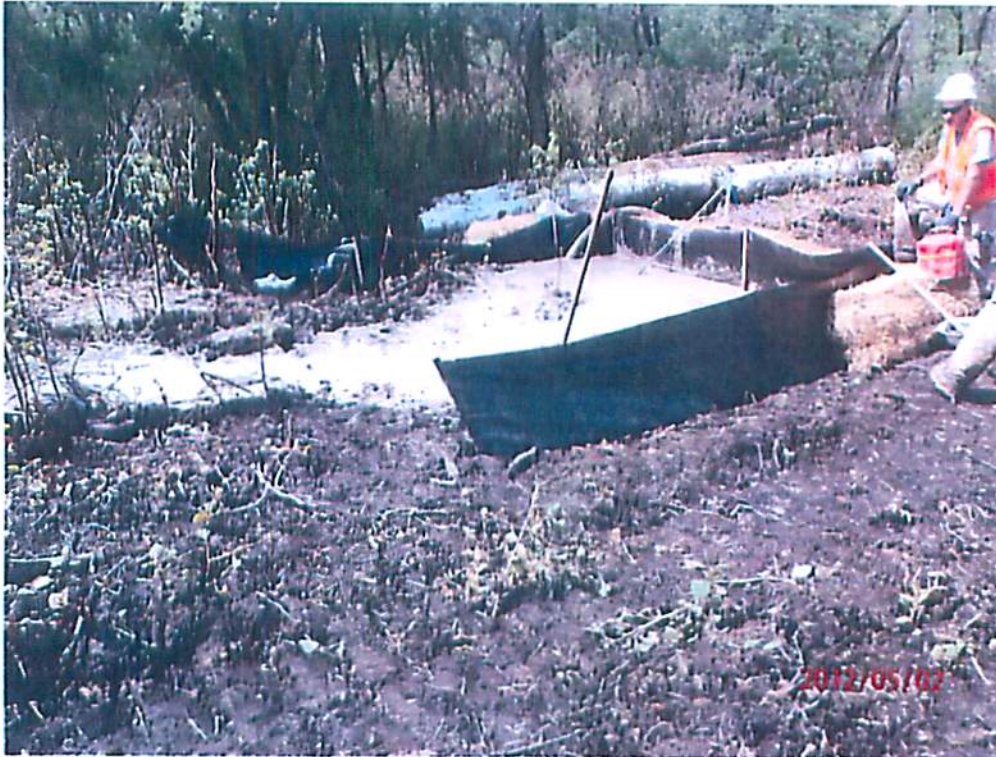
Photo 3. M3 Monongahela River HDD containment.
