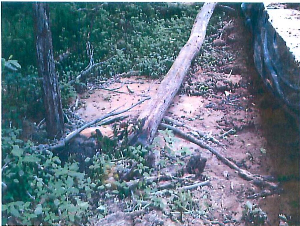
Photo 10. Sediment leaving M3 project site into Jake Run, a violation of State Code 47CSR2-3.
