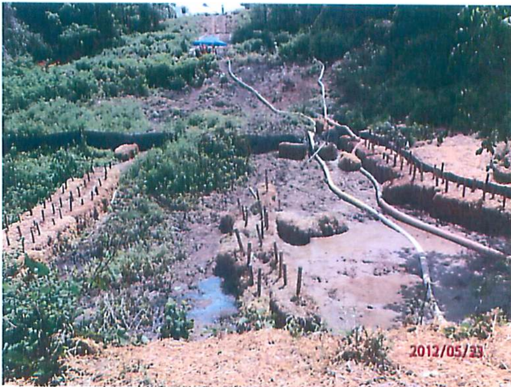
Photo 4. M3 Monongahela River HDD activity with additional release.
