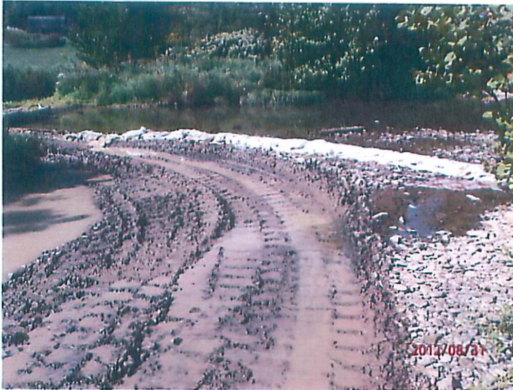
Photo 15. Containment around ingress to inadvertent release sites on Dunkard Creek.
