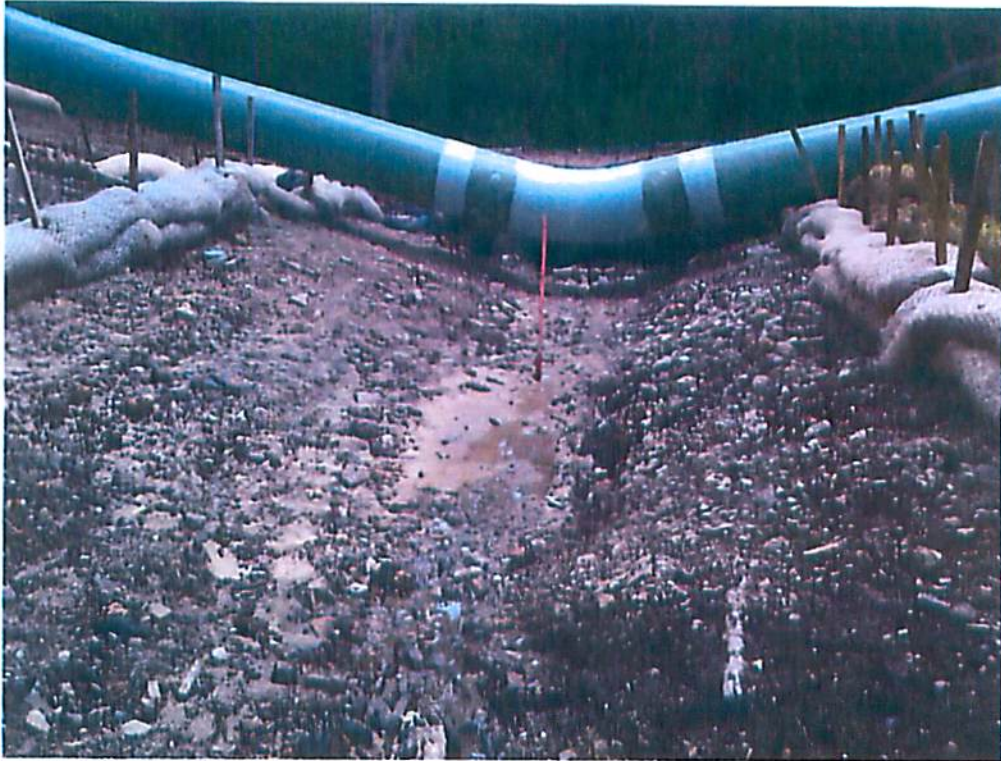
Photo 7. M3 stream crossing of Jake Run in Monongalia County.
