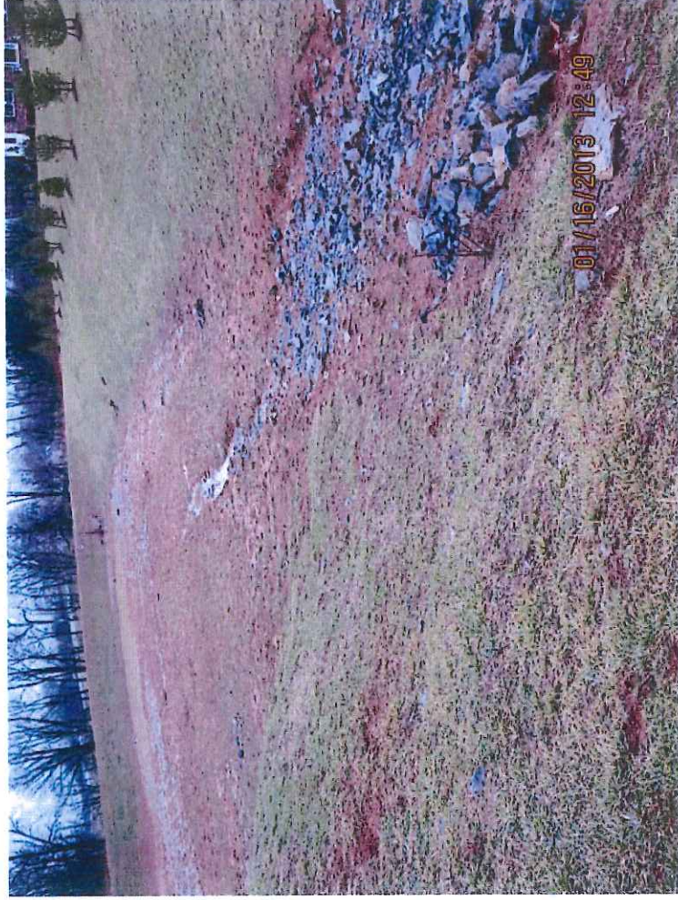
No fore bay in basin "A." Active erosion in bottom of basin.
