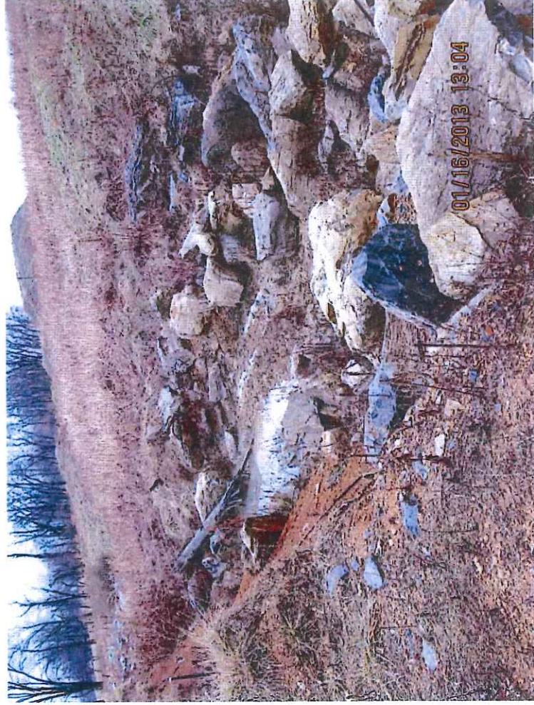
No fore bay in basin "A." Active erosion in bottom of basin.
