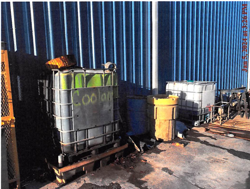
01/05/24 Containers with product did not have adequate secondary containment.
