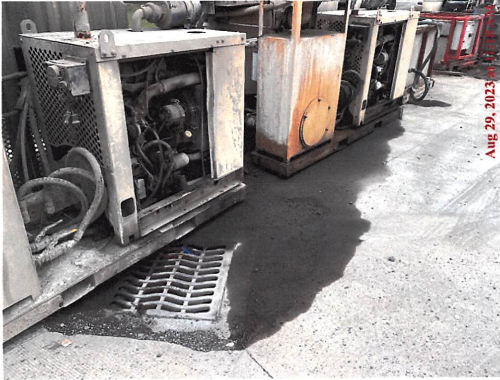
08/29/23 Petroleum product spilling into storm drain that discharges to waters of the State.
