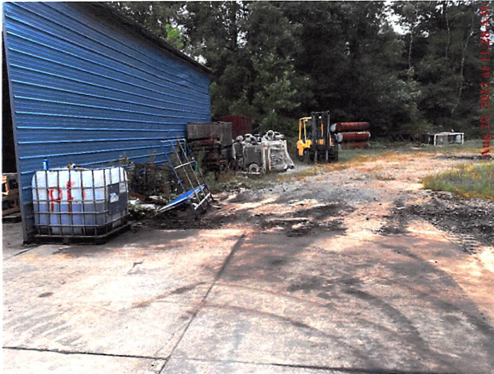
08/29/23 Petroleum staining and tote with product and without secondary containment.
