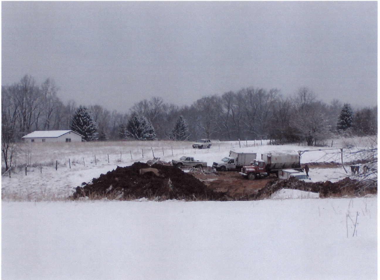
Blasting Operations Relative to Structure #PAT180
