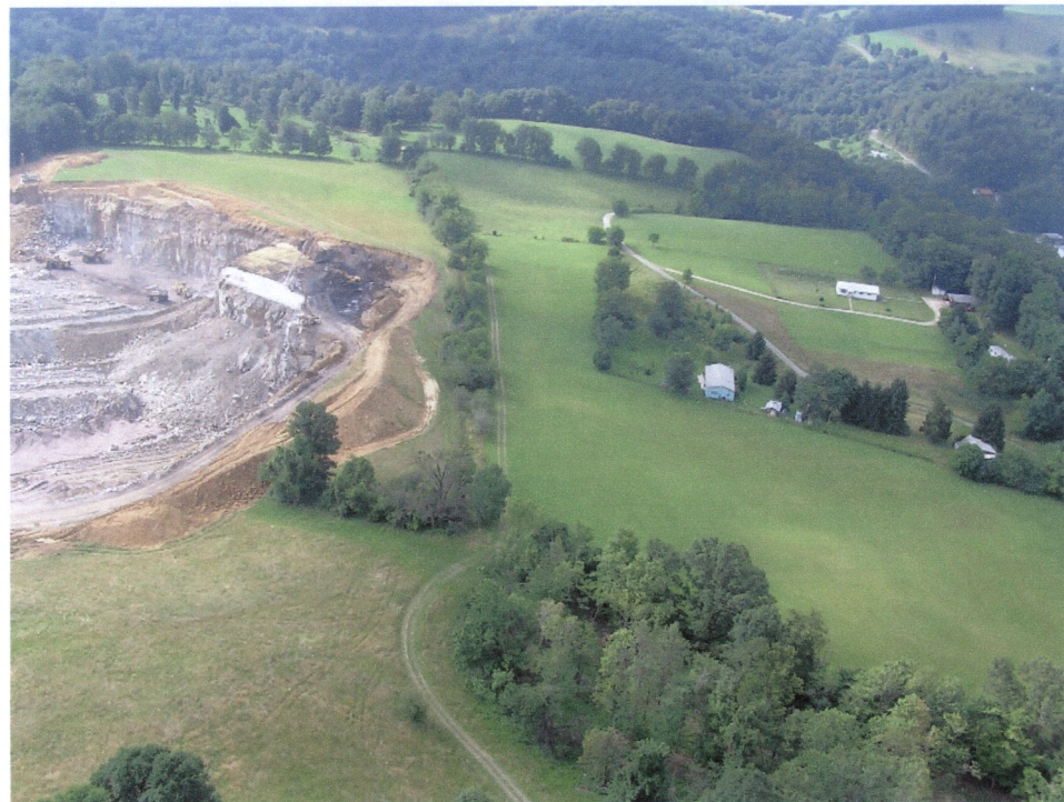
Aerial View Structure#PAT178 and #PAT180 Relative to Blasting Operations
