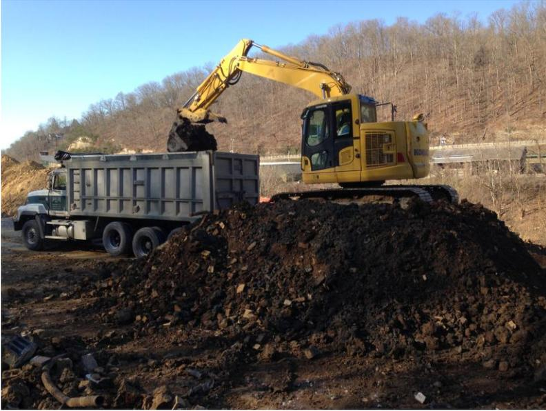
**Figure 6 – A truck being filled with the stockpiled soil and C & D mix with a dark-color stain due to petroleum content. One could smell the petroleum product with some help from the wind.**
