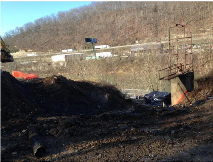
**Figure 5 - A further close-up view of the excavation on Areas 3 and 4, showing a deep cut into the site. An inactive gas line (in the center) came out during the operation**
