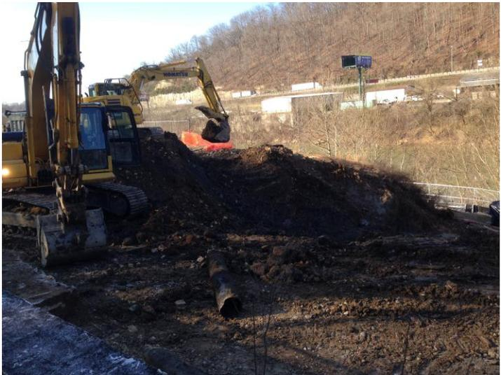
**Figure 4 – A close-up view of the excavation on Areas 3 and 4. An inactive gas line (in the center) came out during the operation**
