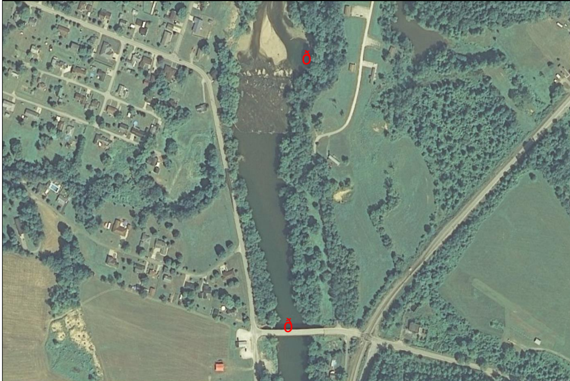
Figure 88. 2003 Aerial Photo of the KC-(11.6) Coal River Ambient Sample Site at Tornado, WV.
