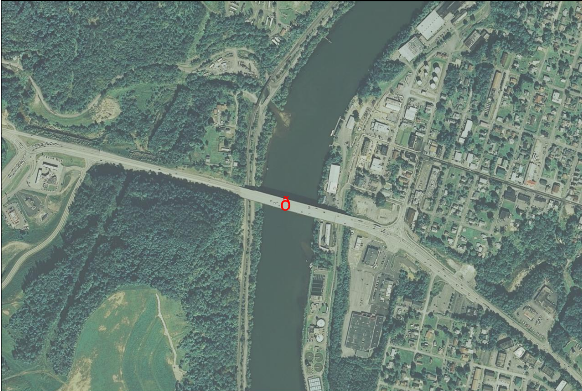
Figure 101. 2003 Aerial Photo of the M-(99.4) Monongahela River Ambient Sample Site in Star City, WV.
