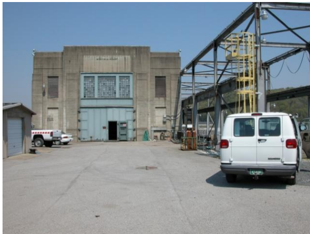
Figure 84. Photo of the Winfield Locks & Dam.
