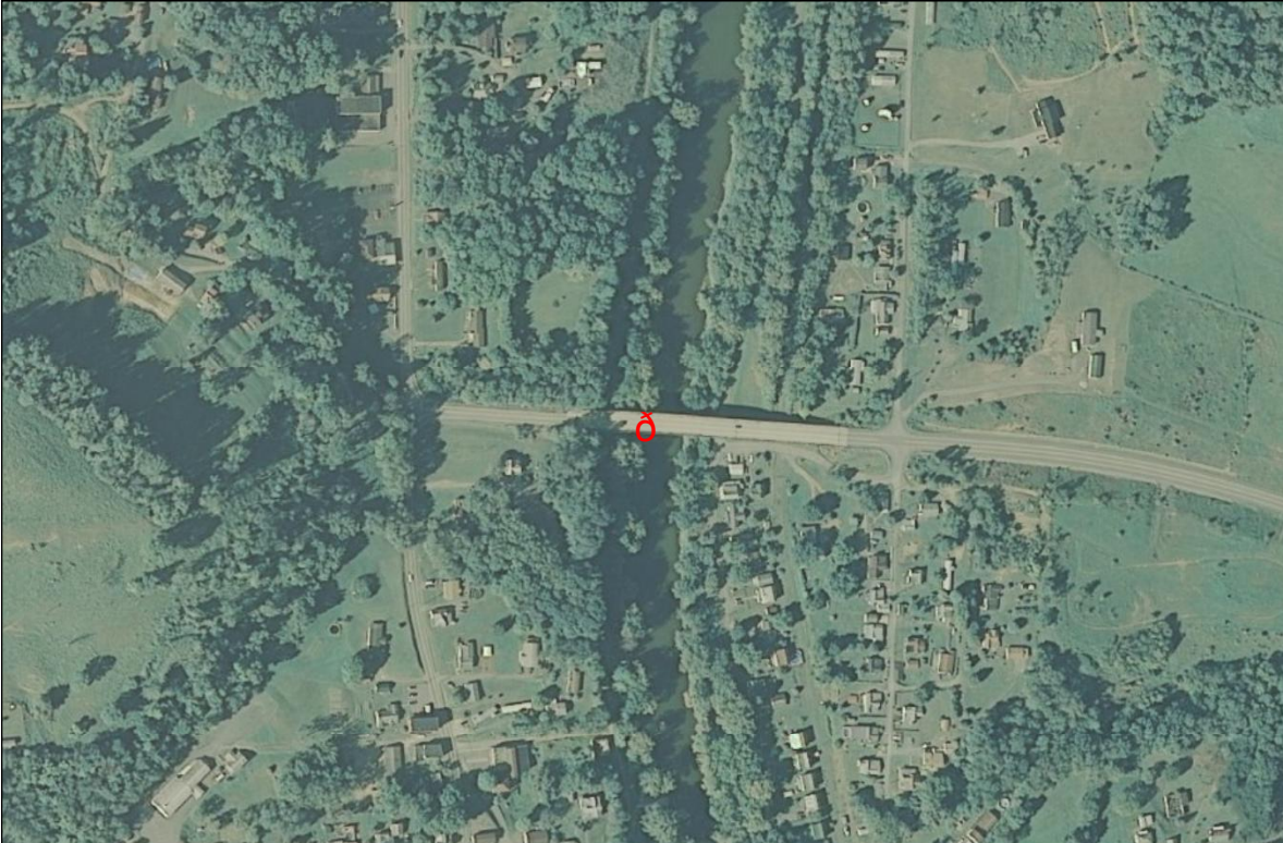
Figure 104. 2003 Aerial Photo of the MW-(12.0) West Fork River Ambient Sample Site at Enterprise,
