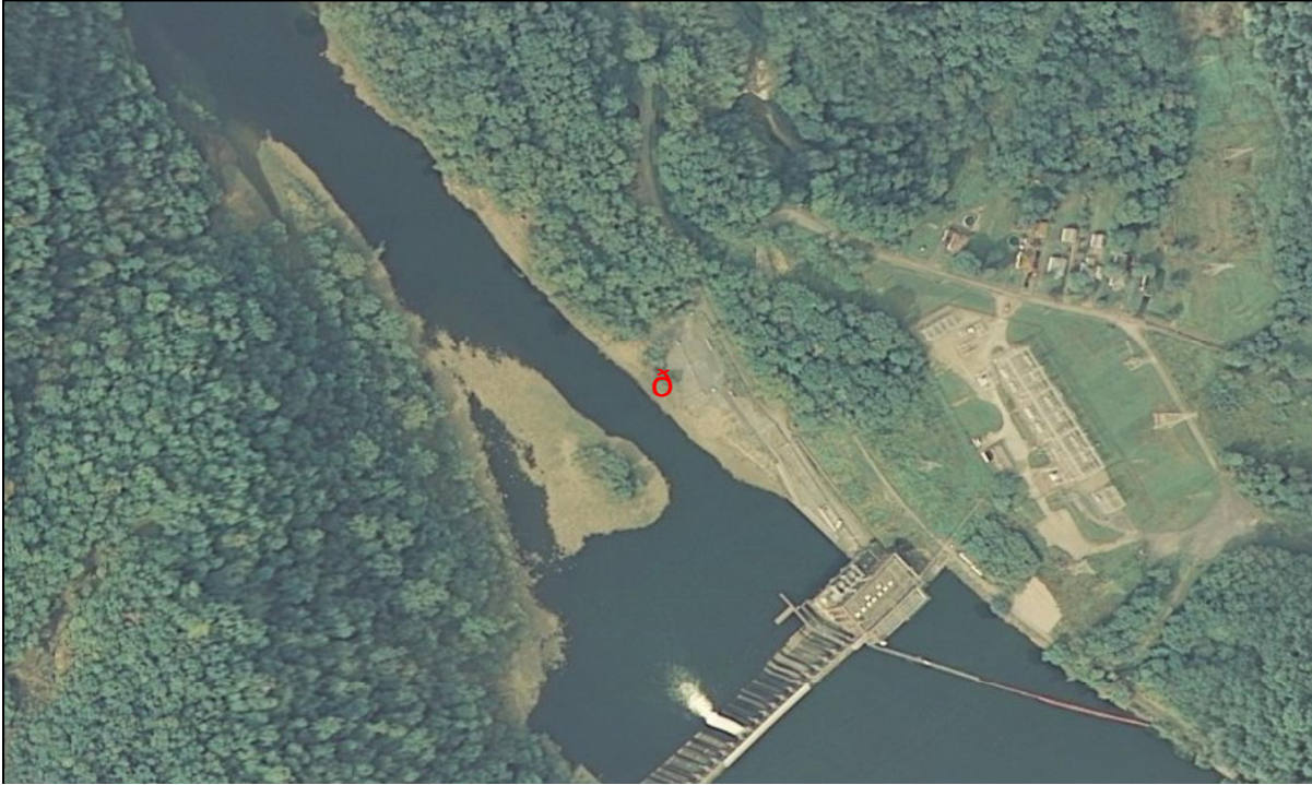
Figure 105. 2003 Aerial Photo of the MC-(3.5) Cheat River Ambient Sample Site in Lake Lynn, PA.
