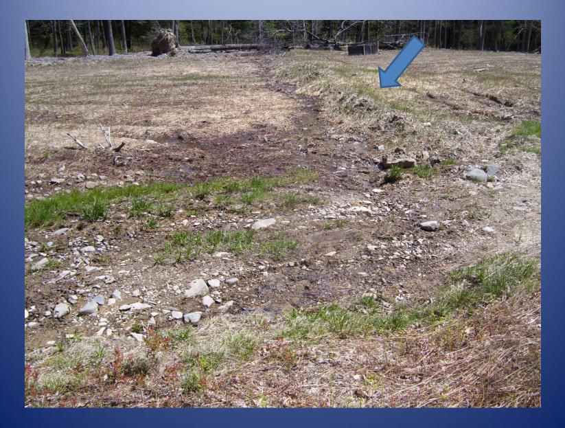
Slope breakers must go entirely across the ROW to ensure the water does not come back across the ROW needed
