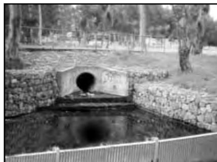
Stormwater filters such as shown here are designed to catch litter that might accumulate in other areas.
