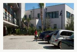
Permeable Paving materials include concrete, asphalt, and interlocking pavers that allow runoff to filter through voids into a gravel storage reservoir.
