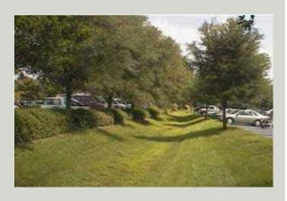
Grass Swales are designed as conveyance systems with enhanced design features to also provide a level of stormwater treatment and retention.
