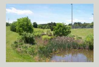
Constructed Stormwater Wetlands are shallow vegetated depressions with multiple cells of varying depths. Stormwater wetlands are not considered a runoff reduction practice, but can be used for water quality treatment and, in some cases, to meet stormwater detention requirements.
